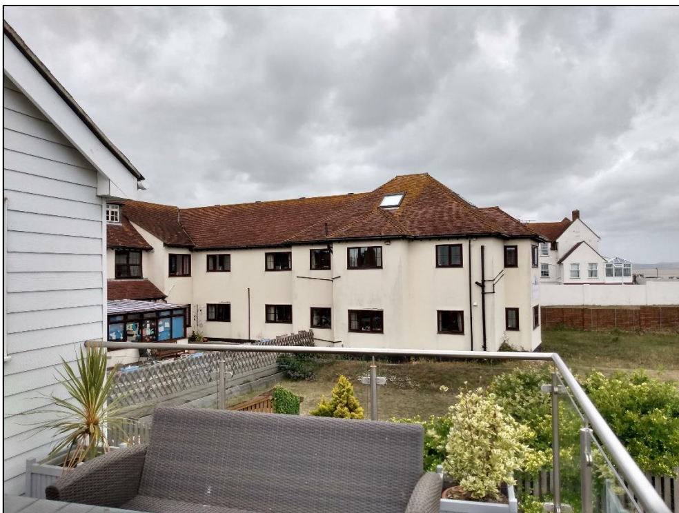
Fig.6 Flank view from balcony of The Coast House (to south)
