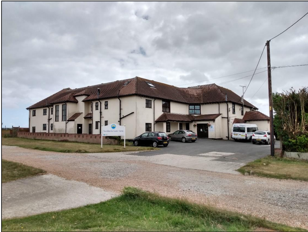
Fig.5 View from St Andrew's Road
